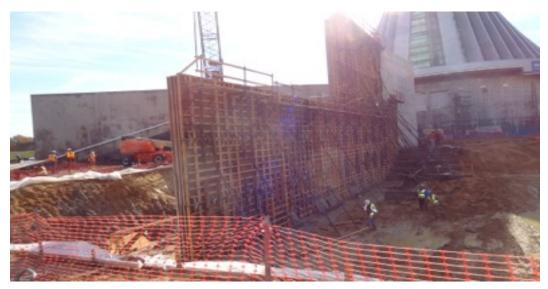
While this work is in progress, new exhibit space interior concrete walls are being poured that will separate the new exhibit galleries and I -Max Theater. Once the old walls have been removed and the new galleries built, a new exterior wall and roof will be built over the exhibit space, the roof will the covered with soil and grass to match the other side of the museum. (Photo by David H. Hugel)
